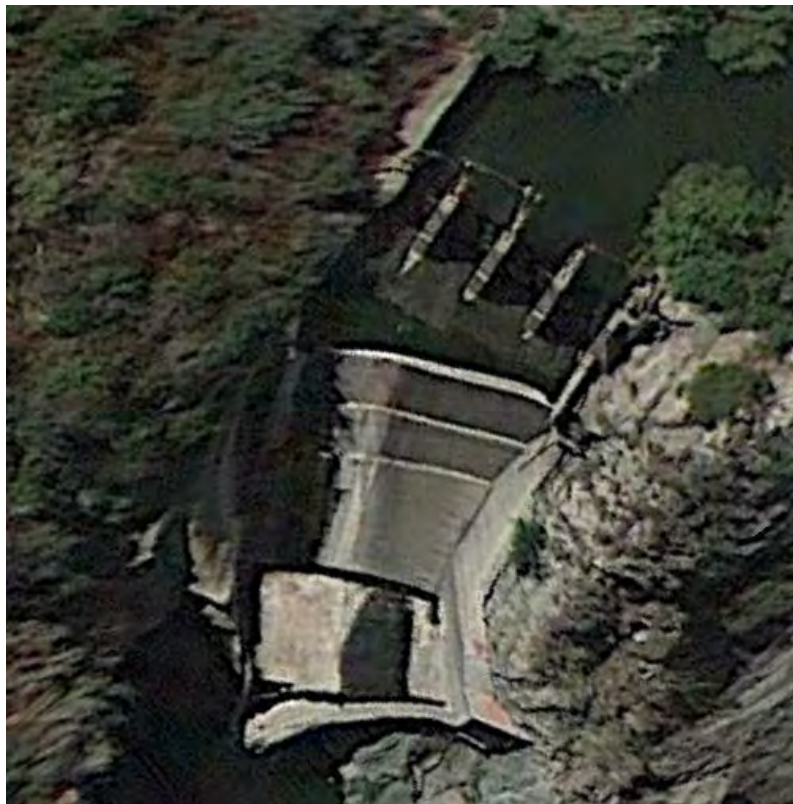
Figure 2.5-1 Rindge Dam Spillway
