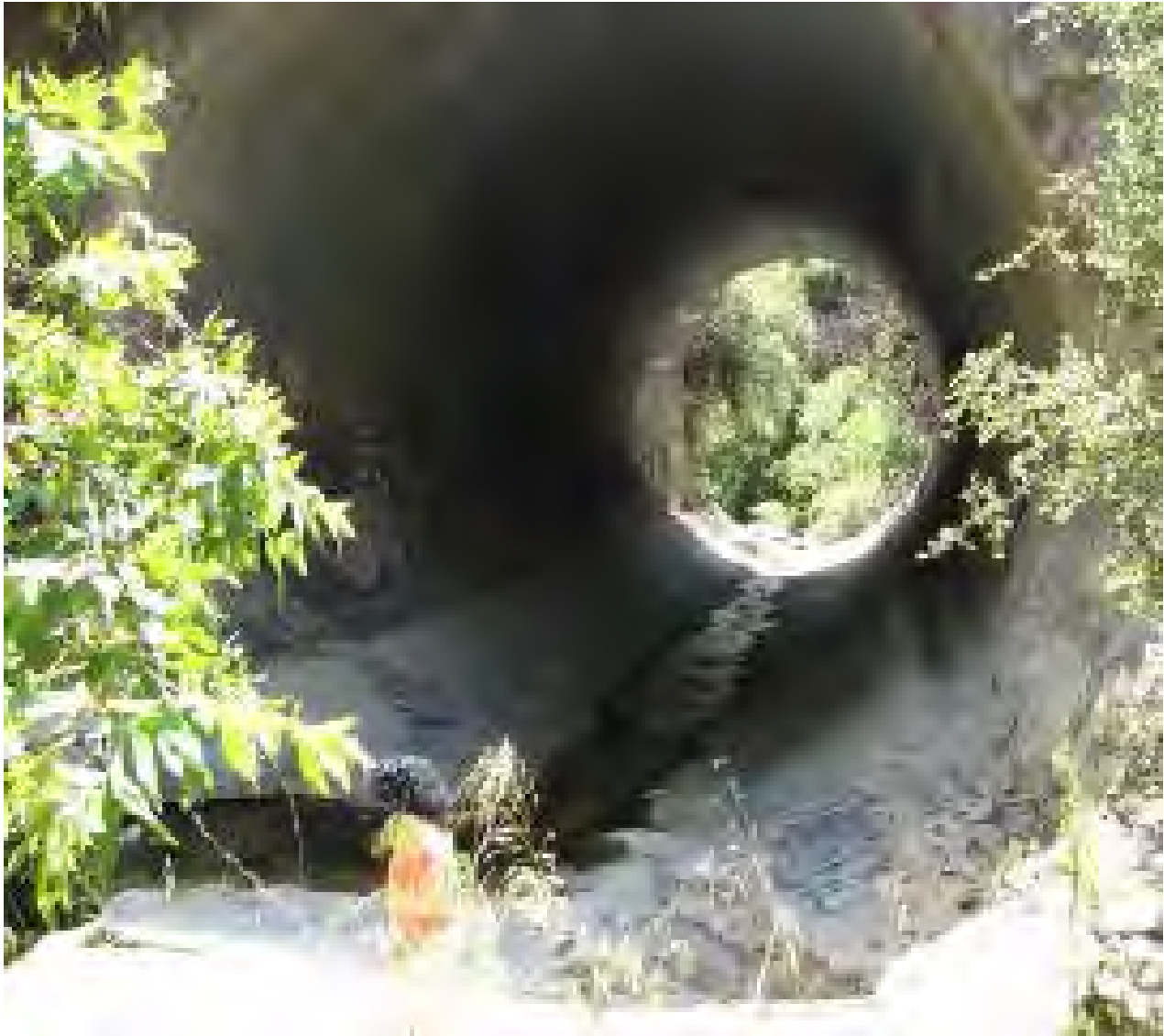
6 7 Figure 3.8-2 CC5, Cold Canyon Road Culvert (Picture taken looking upstream)
