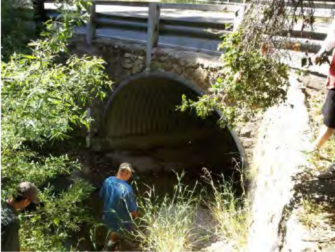
Figure 3.4-2 CC1, Piuma Culvert (Picture taken looking upstream)
