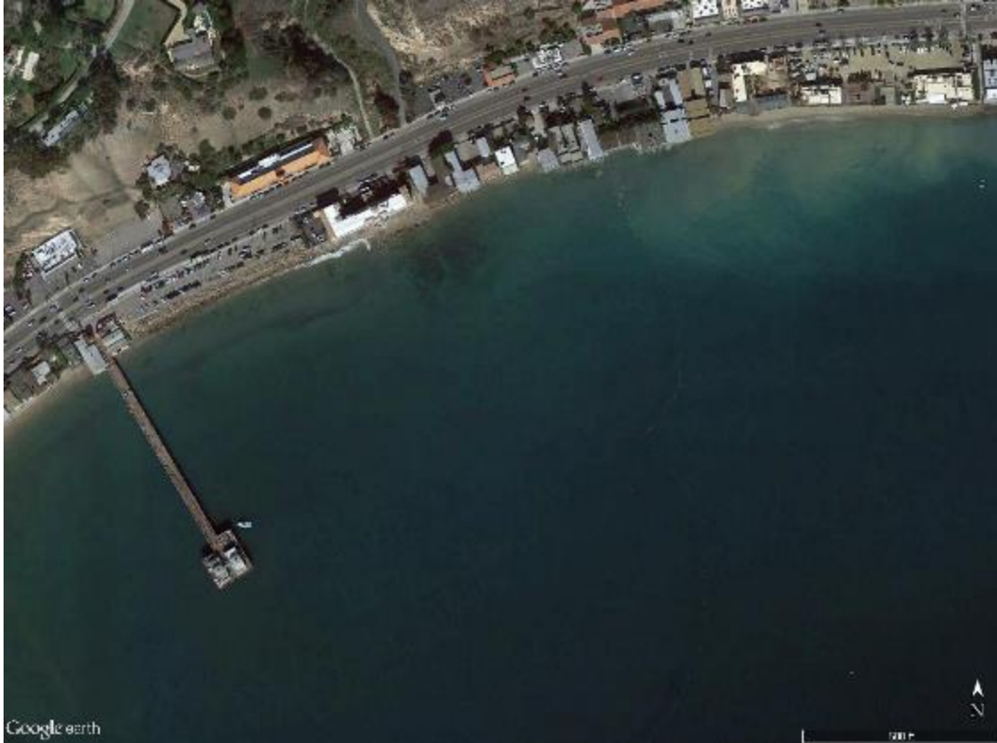
1 2 Figure 4.3-3: Present condition of shoreline near Malibu Pier (Google, 2016)
