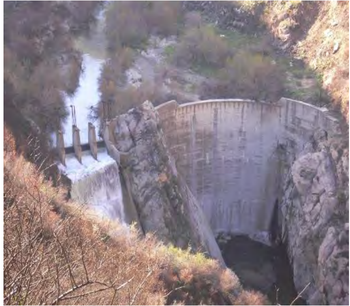
Photo 1.10-1 – Rindge Dam Arch & Spillway
