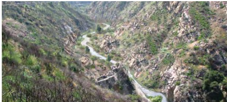
Figure 4.10-1 - Former Rindge Dam Site - Post Construction
