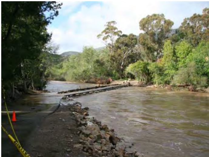
Photo 4.4-12 - Cross Creek Rd. Bridge after Storm
