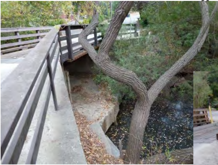
Photo 4.4-3 - Photo 4.3 - CC2 Bridge & Concrete Apron
