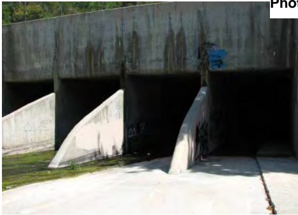
Photo 4.4-8 - LV3 Concrete Apron
