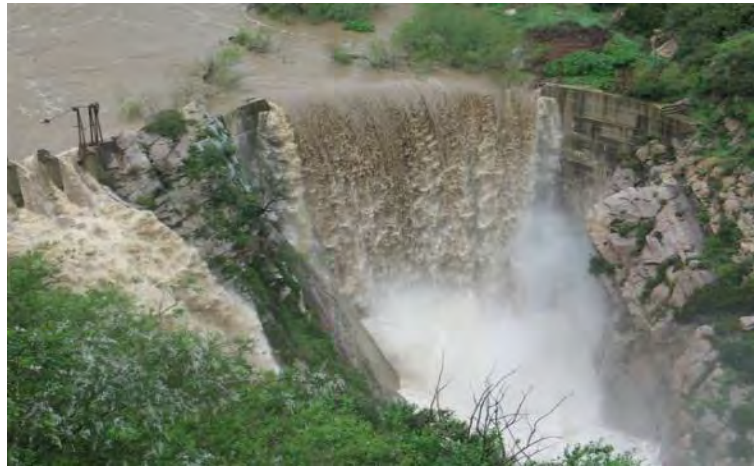
Photo 4.4-10 - Rindge Dam 2005 Storm
