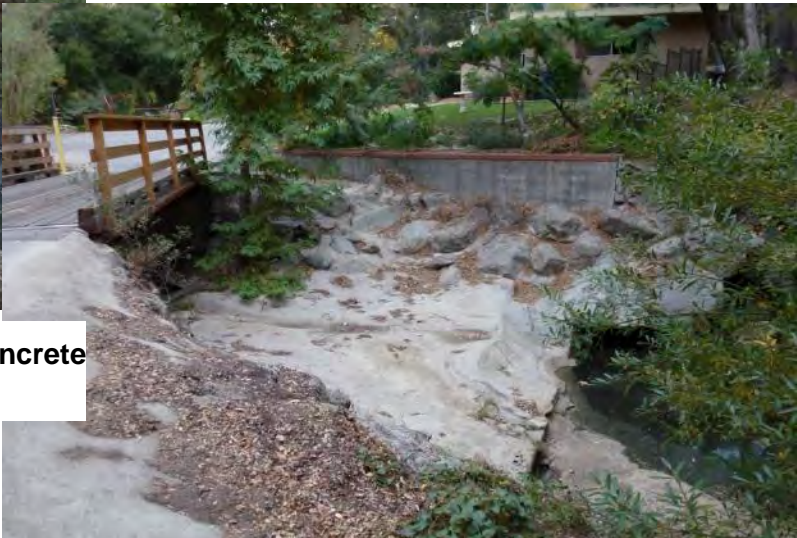
Photo 4.4-4 - CC3 Bridge & Concrete Apron
